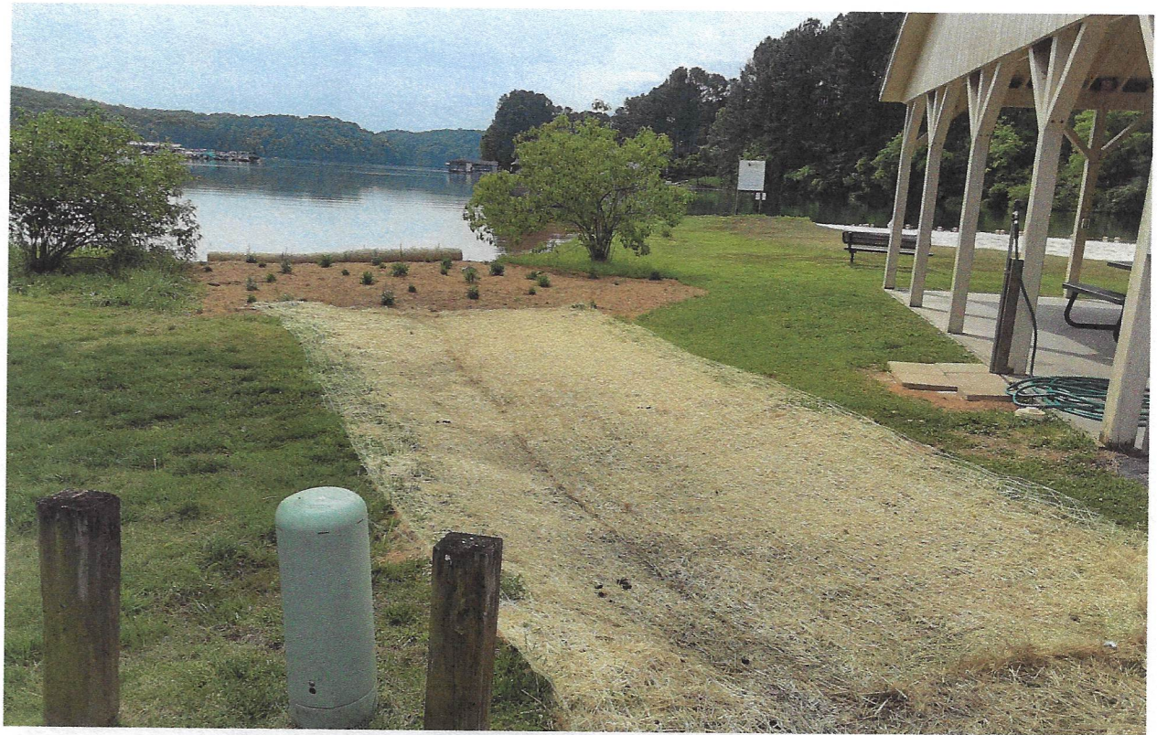
Construction of Rain Garden (drainage swale leading to inlet to lake (2023)
